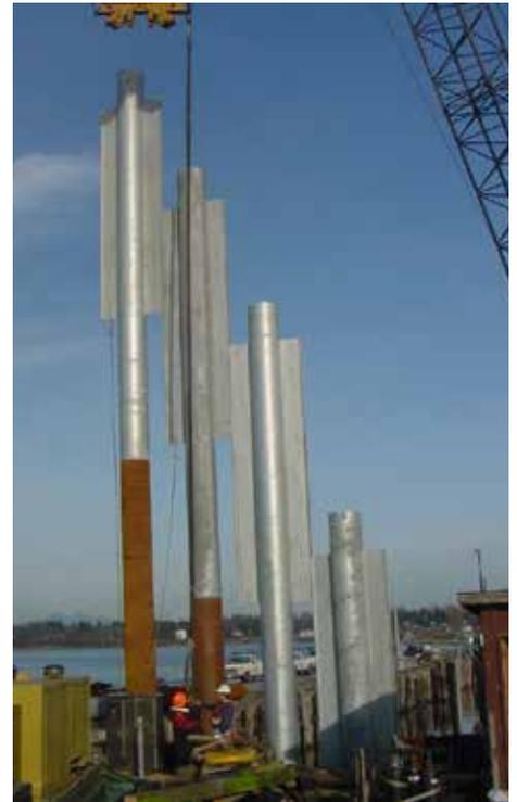
the pipe piles) corkscrewed the wave barriers during difficult driving and also provided uplift resistance against wave action.
